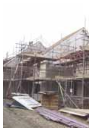
Timber frames are erected
